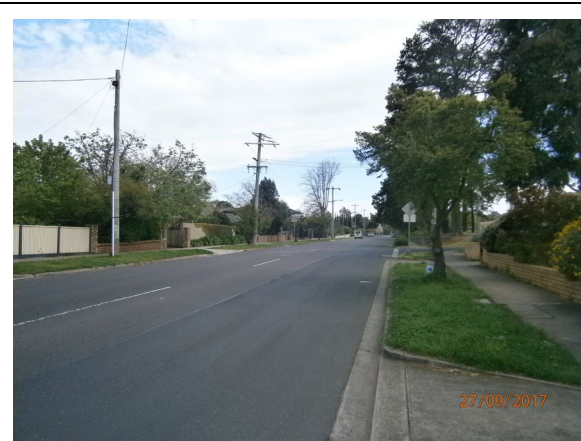
Figure 4: The Boulevard – View West
